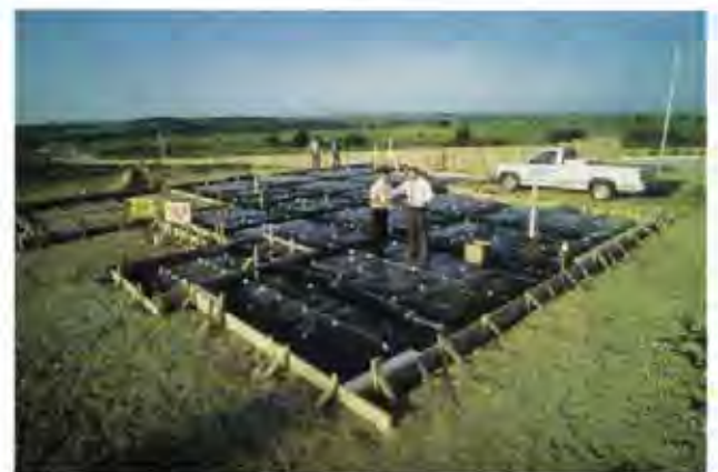
Fig. 2.71 Residential Ribbed Foundation Courtesy of Jack W. Graves Jr., GSI Post-Tension
