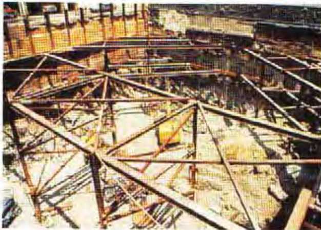
Fig. 15.1 Conventional Diagonal Bracing Courtesy of Schnabel Foundation Company
