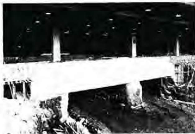
Fig. 2.58 Excavations Under Transfer Girders Supported on Original Caissons, O'Hare International Airport, Chicago, IL
