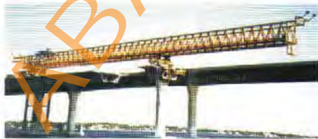
Fig. 12.50 Erection Truss for Cantilever Construction
