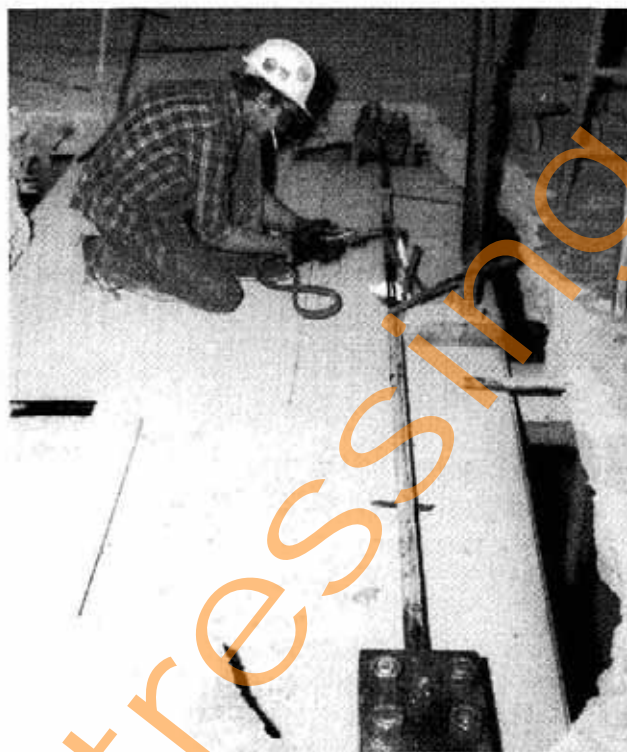
Fig. 6.27 Procedure for De-Tensioning Tendons at Stairwell Opening
