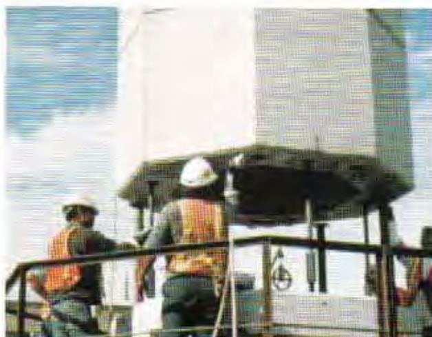
Fig. 12.75 Erection of Segments for a Precast Segmental Concrete Bridge Pier
