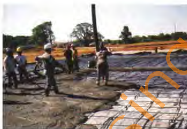
Fig. 2.72 Residential Uniform Thickness Slab-on-Ground
