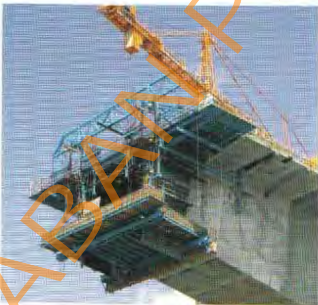
Fig. 12.41 Cantilever Construction: Travelers and Formwork for Segments Courtesy of VSL
