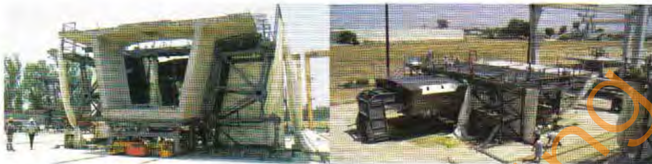
Fig. 12.49 Formwork for Match-Casting of Precast Concrete Segments Courtesy of Hilliard Bond
