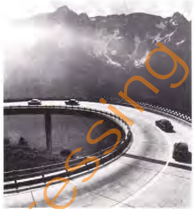
Fig. 12.2 Cast-in-Place Post-Tensioned Bridge, Switzerland Courtesy of BBR International
