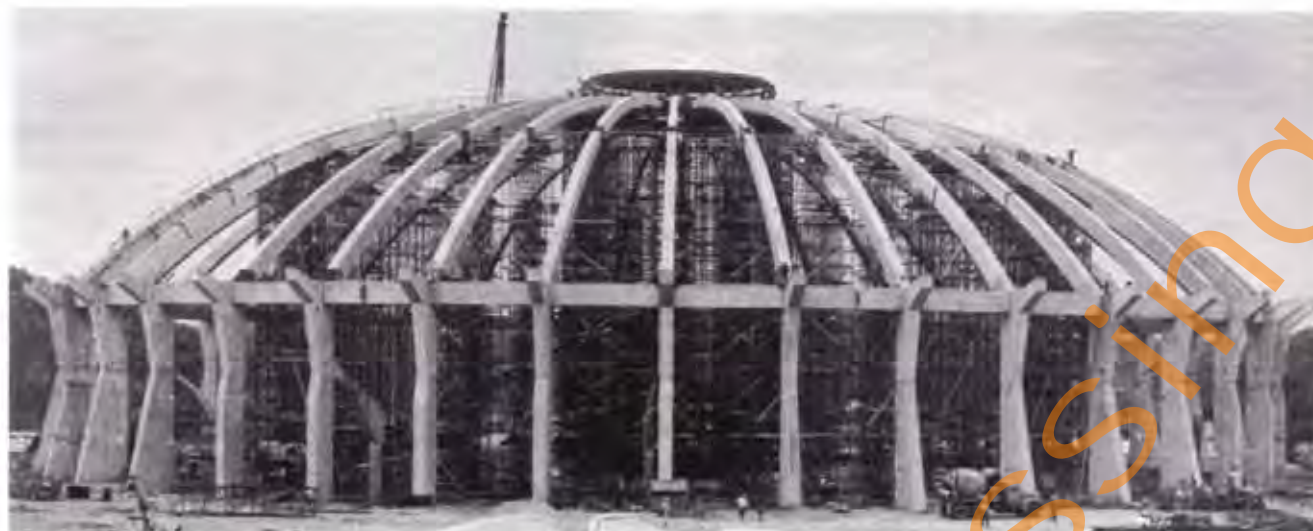
Fig. 2.63 Construction of Domed Field House, University of West Virginia Field House, Morgantown, WV
