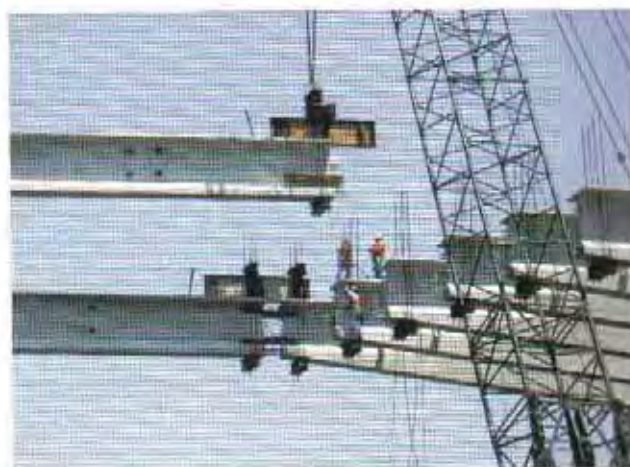
Fig. 12.34 Spliced I-Girder Bridge
