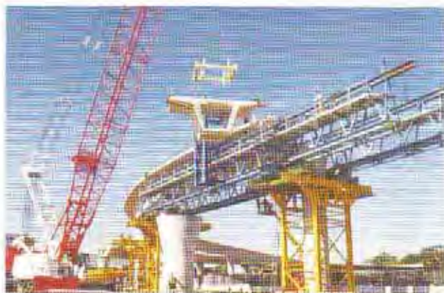
Fig. 12.52 Under-Slung Erection Girder
