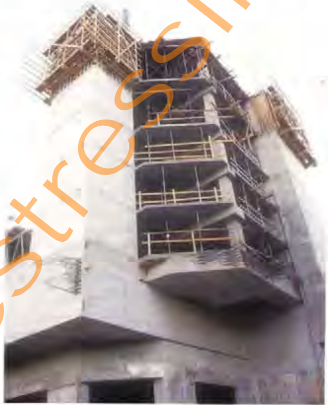
Fig. 9.3 Post-Tensioned Transfer Beam Courtesy of Ken Bandy
