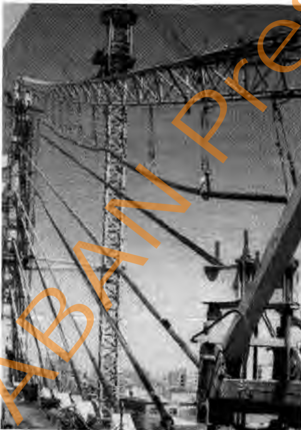
Fig. 13.19 Cable Erection With Spreader Bars Courtesy of DYWIDAG-Systems International, USA
