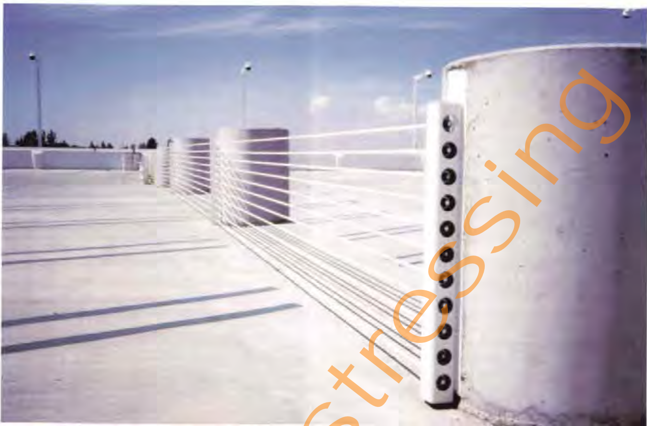
Fig. 2.84 Barrier Cables in Nike Parking Garage Courtesy of Cary Kopczynski & Company, Inc.
