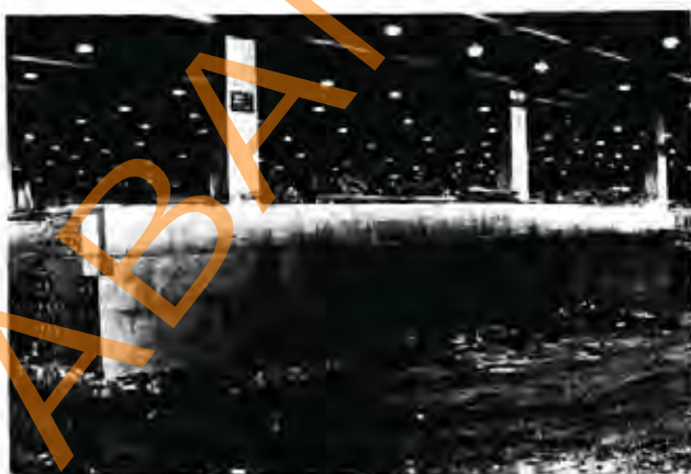
Fig. 2.57 Completed Transfer Girder, O'Hare International Airport, Chicago, IL
