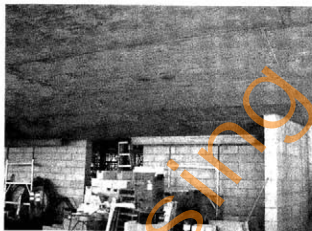
Fig. 6.26 Tendon Locations Marked at Bottom of Slab by Use of Spray Paint on the Form Prior to Concrete Placement Courtesy of Seneca Structural Engineering, Inc.
