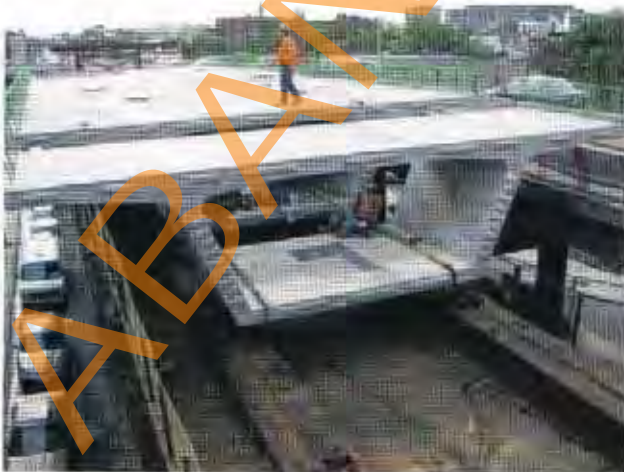
Fig. 12.18 Single-Cell Box Girder
