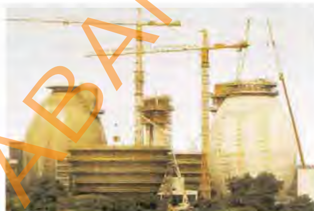
Fig. 2.49 Egg-Shaped Sludge Digester Tanks, Bottrop, Germany Courtesy of VSL
