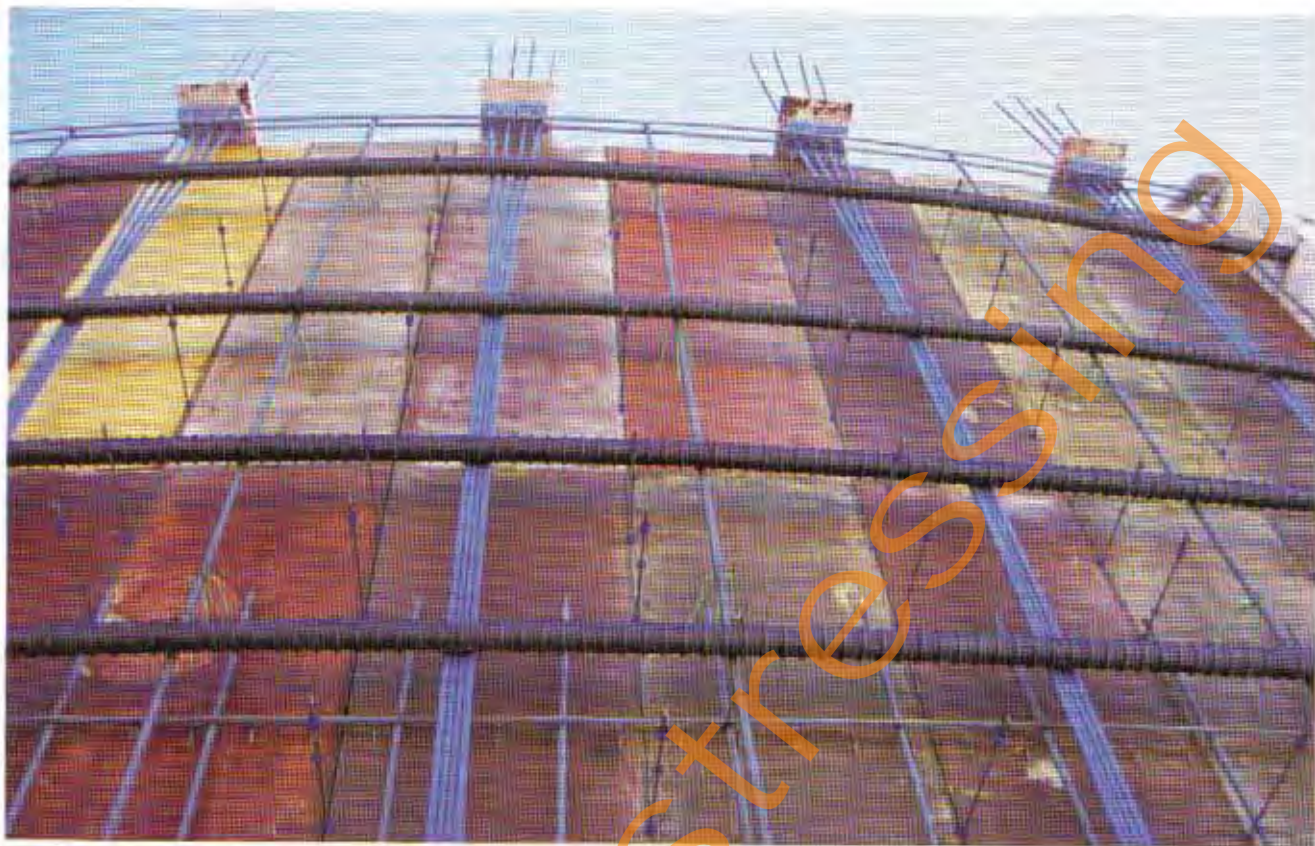
Fig. 14.9 Typical Distribution of Tendons in a Tank Wall Courtesy of Jorgensen & Close Associates, Inc.
