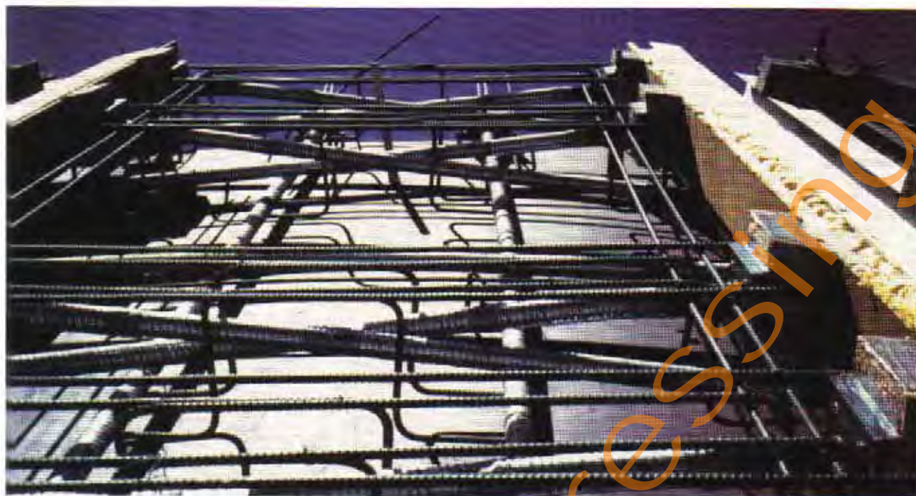
Fig. 14.14 Tendon Intersection at a Buttress
