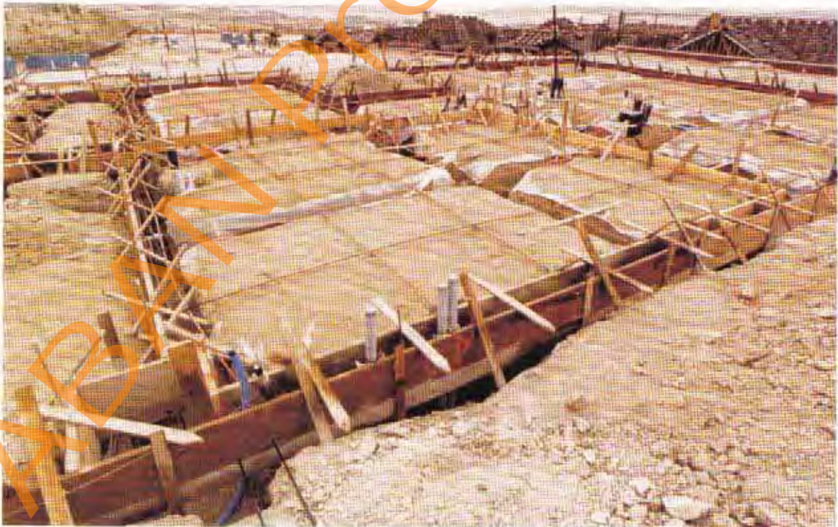
Fig. 11.1 Ribbed Foundation
