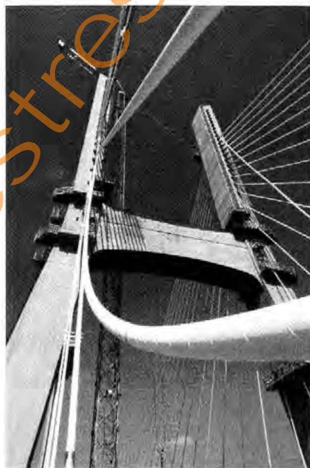
Fig. 13.12 Surface Contours on Cable Sheathing, Tagun Bridge, Portugal Courtesy of Freyssinet International
