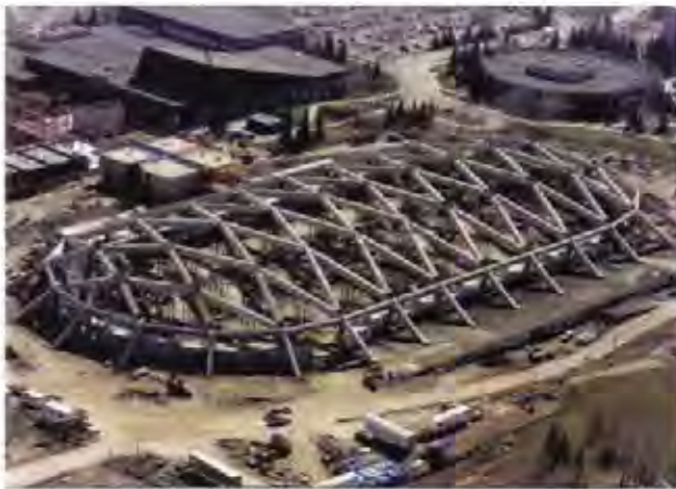
Fig. 2.54 Precast, Post-Tensioned Arch Roof Construction of The Calgary Olympic Oval
