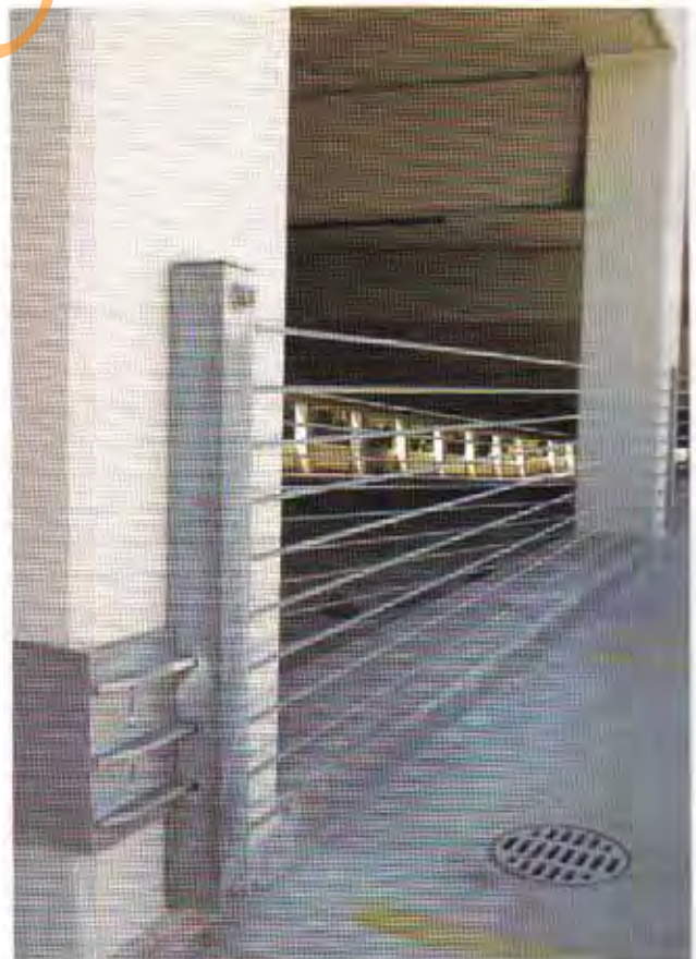
Fig. 10.6 Barrier Cable
