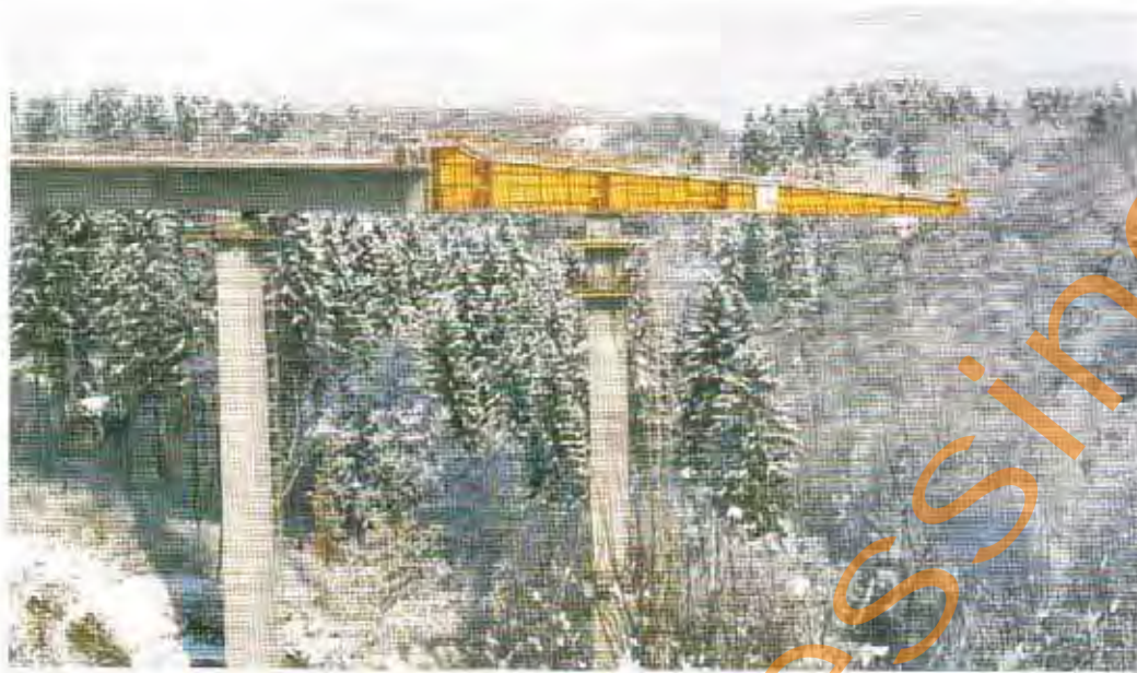
Fig. 12.65 Launching Nose Courtesy of Norbert Luksch
