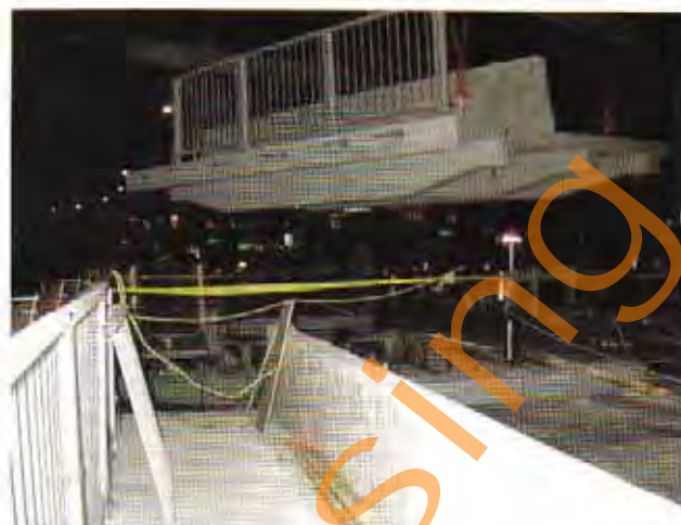
Fig. 12.76 Precast, Post-Tensioned Dock Panels for Rehabilitation Courtesy of The Jacques-Cartier and Champlain Bridges Inc.
