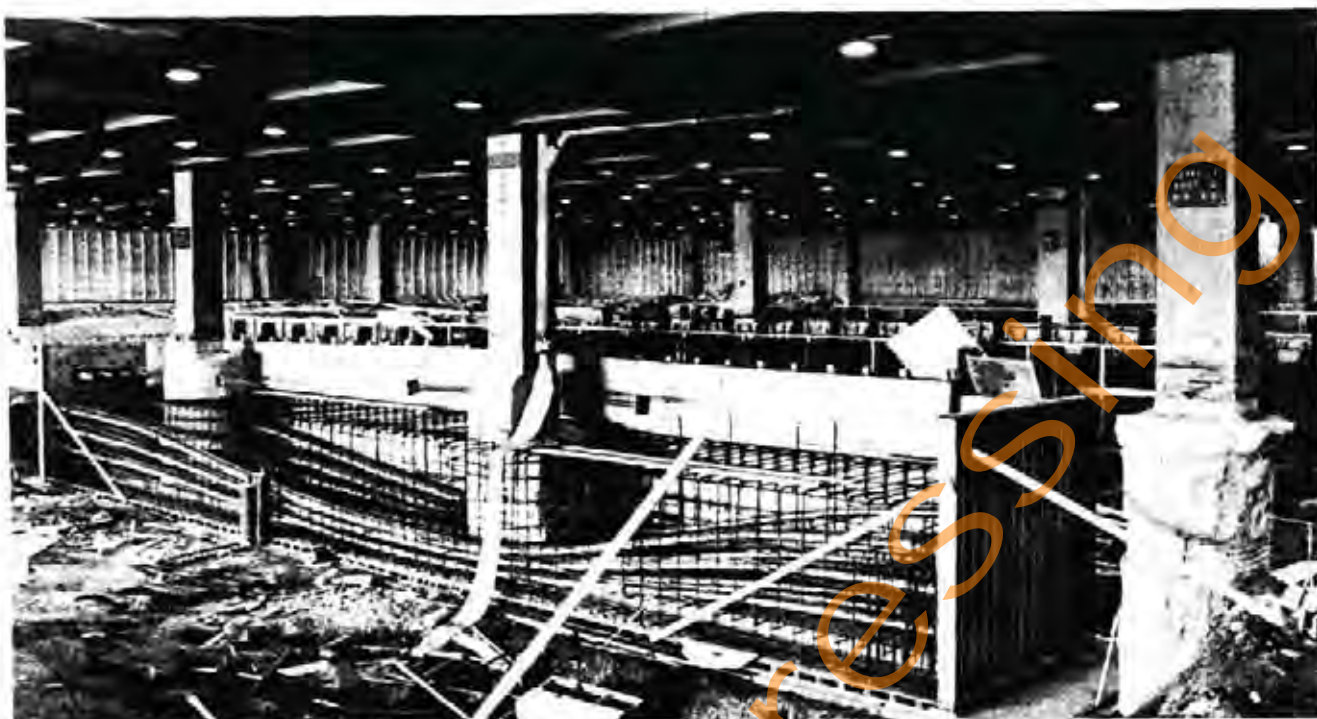
Fig. 2.56 Transfer Girder Construction, O'Hare International Airport, Chicago, IL
