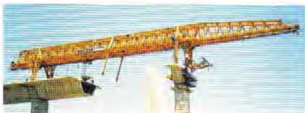
Fig. 12.53 Overhead Erection Girder
