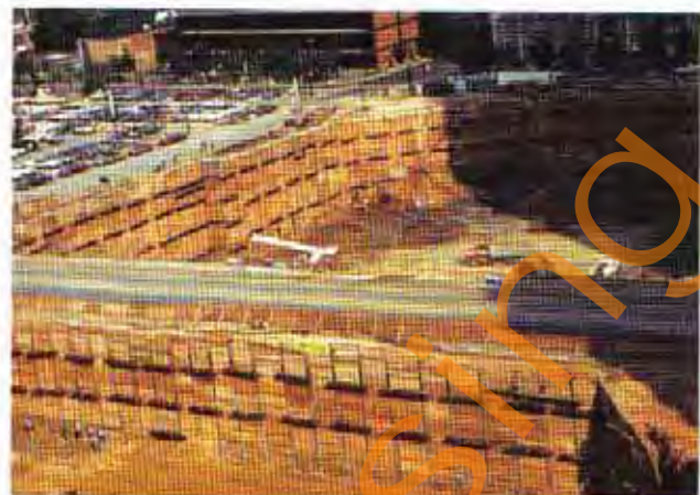
Fig. 15.2 Temporary Tieback Shoring Courtesy of Schnabel Foundation Company
