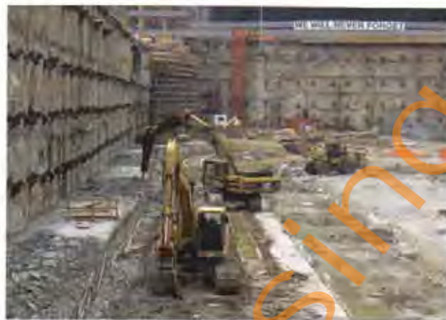
Fig. 2.68 Ground Anchors to Stabilize the Basement for WTC Cleanup Courtesy of DYWIDAG-Systems International, USA
