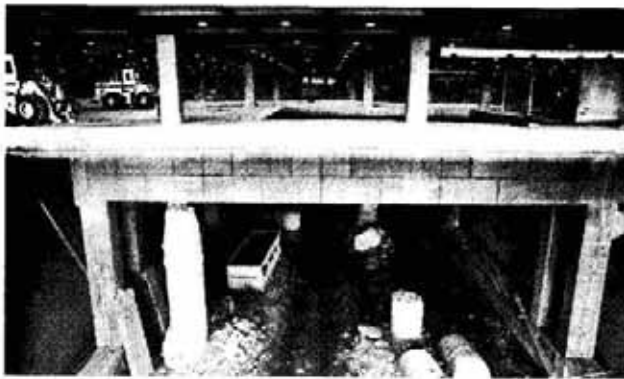
Fig. 2.59 Cutting Off Original Caissons, O'Hare International Airport, Chicago, IL
