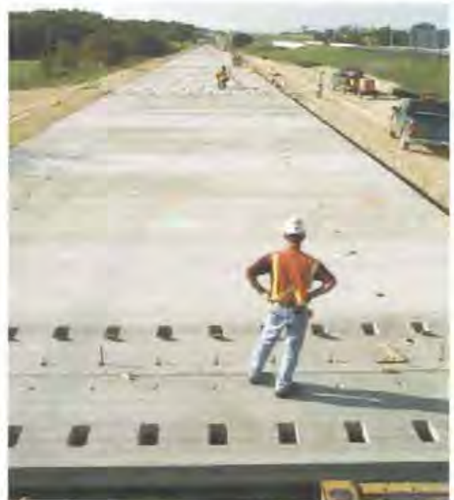
Fig. 2.81 I-35 Frontage Road Precast Pavement, Georgetown, TX Courtesy of DYWIDAG-Systems International, USA
