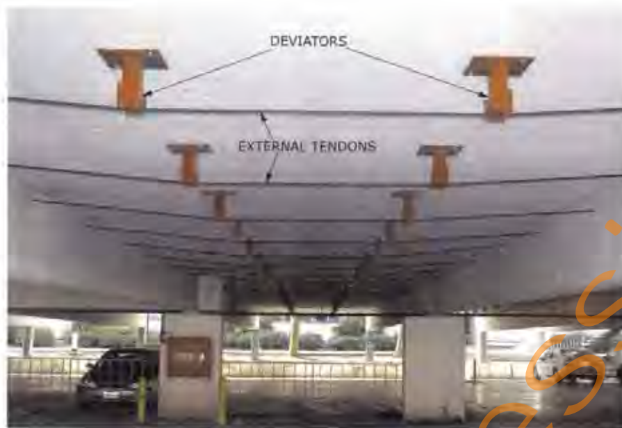
Fig. 3.4 External Tendons in a Retrofit Application Courtesy of Seneca Structural Engineering, Inc.
