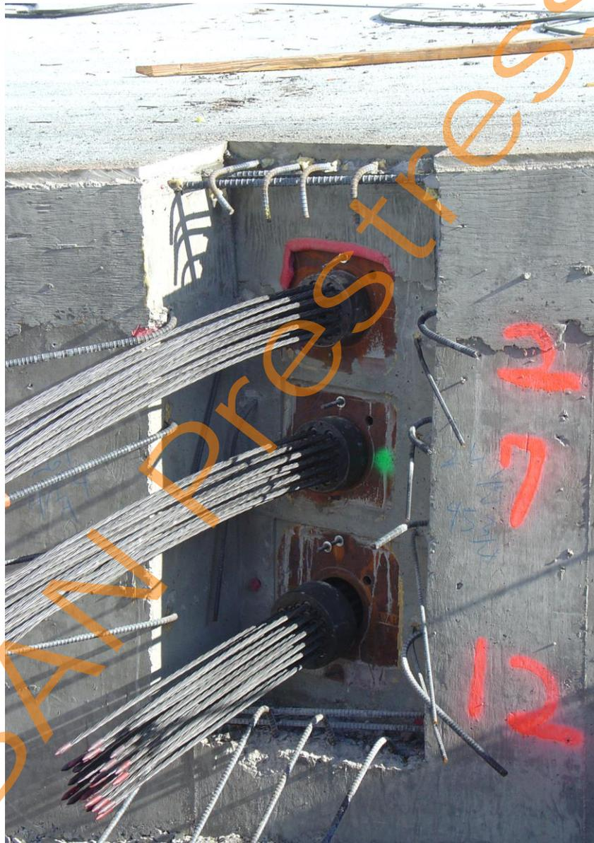
Figure 2.2 Post-tensioning on a highway overpass
