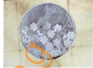
Fig. 3: Properly grouted tendon section
