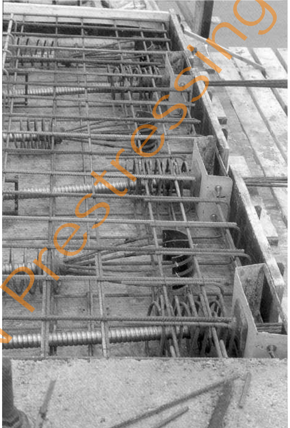
Figure 1.1: Anchorages provide for the safe introduction of post-tensioning forces into the concrete.
