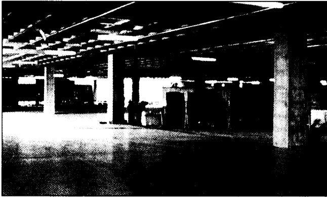
Figure 2.9(e) Windmill Hill, Swindon: post-tensioned waffle slab
