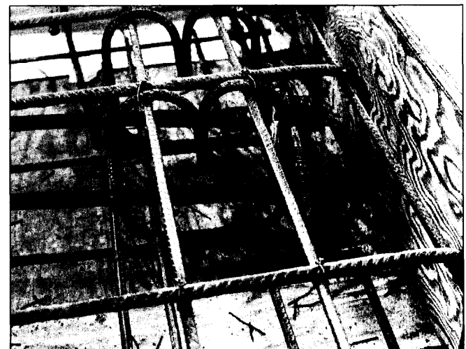
Figure 6.6 Dead-end anchorage
