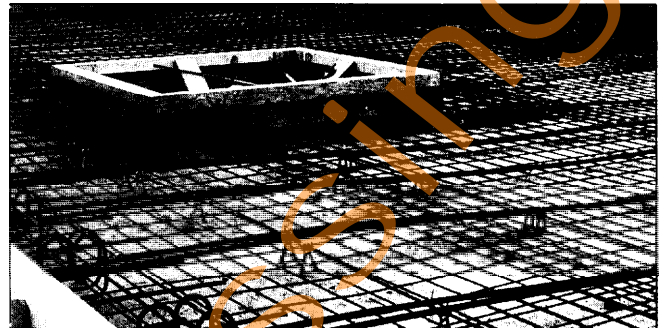
Figure 2.5 Unbonded tendons in a floor slab
