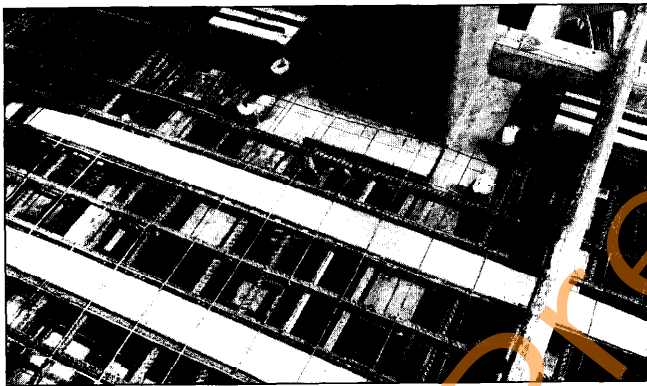
Figure 5.6 Steel shearhead in post-tensioned floor slab
