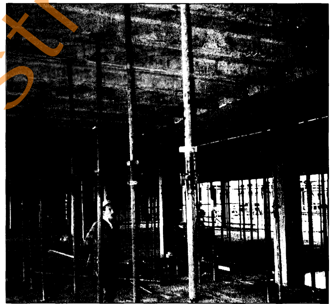
Figure 6.10 Back-propping of post-tensioned ribbed slab
