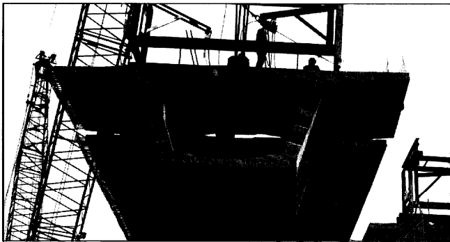
Figure 2.3 Segmental construction in bridge decks
