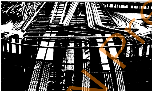
Figure 2.4 Bonded tendons in beam
