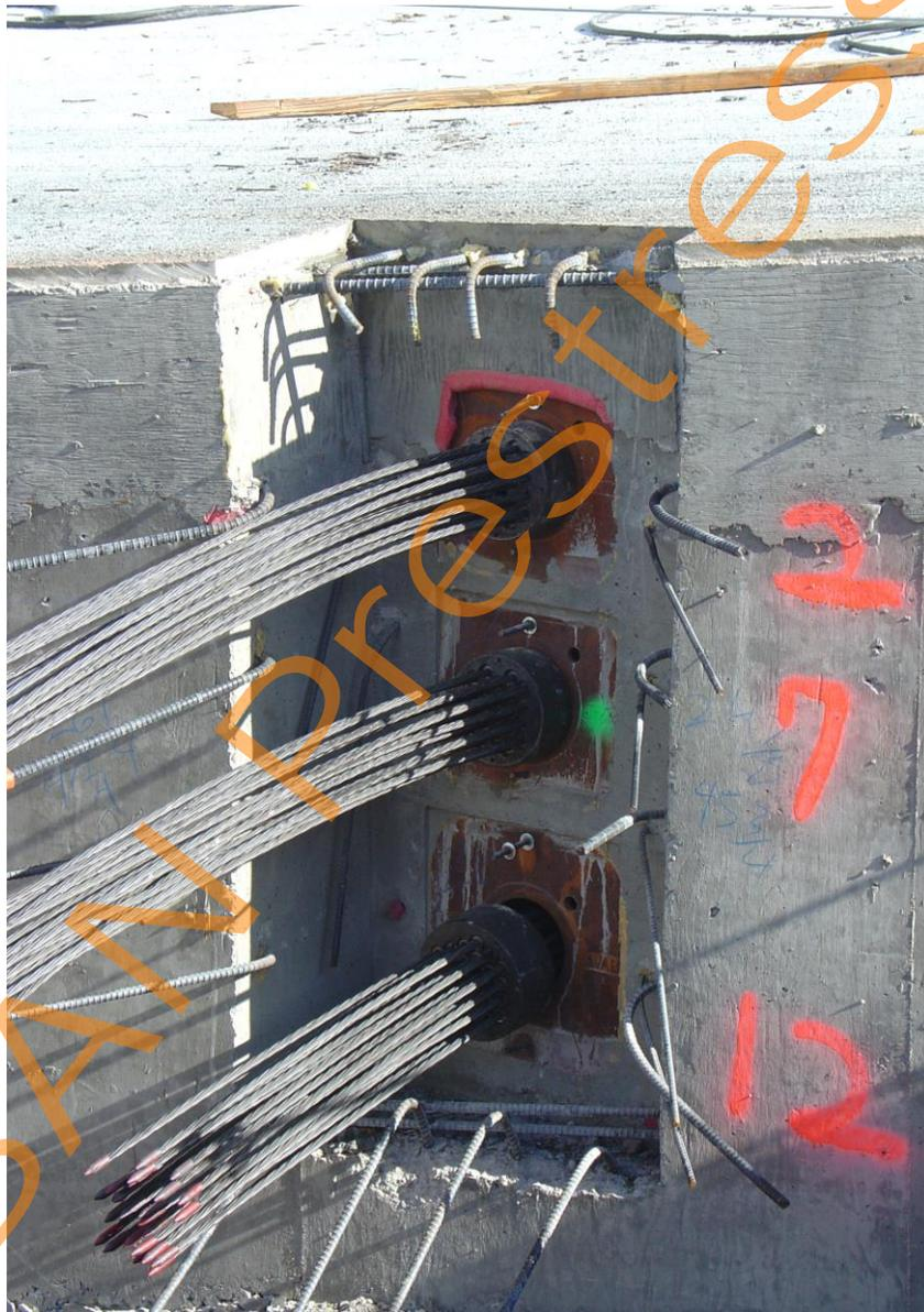
Figure 2.2 Post-tensioning on a highway overpass
