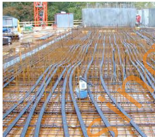
Bonded slab post-tensioning system
