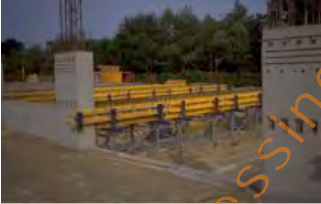
Figure 3.18: Downstand beams in the formwork
