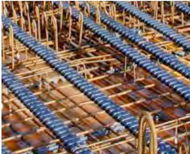
Figure 2.32: Polyethylene flat ducts(PT-Plus TM )
