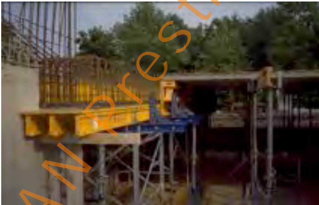
Figure 3.19: Formwork the the downstand beam serves simultaneously as support for the element floors
