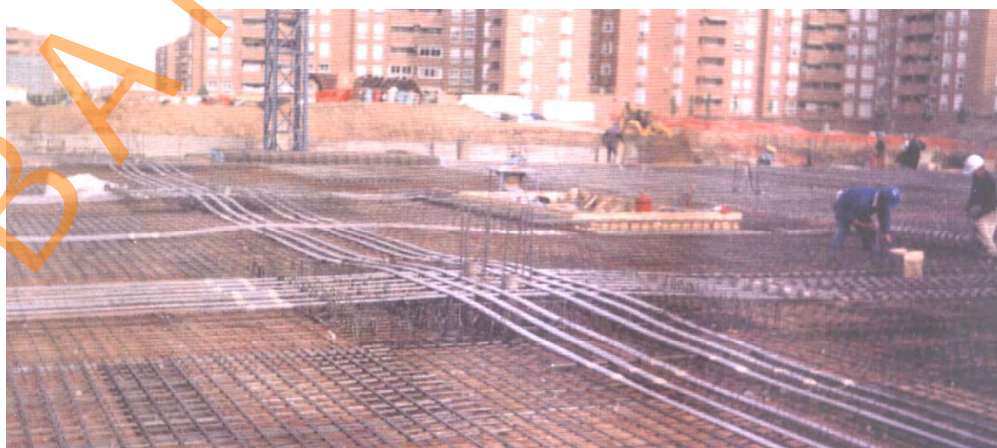
Figure 3.7: View of reinforcement and of the prestressing ducts previous to the concreting of level 1
