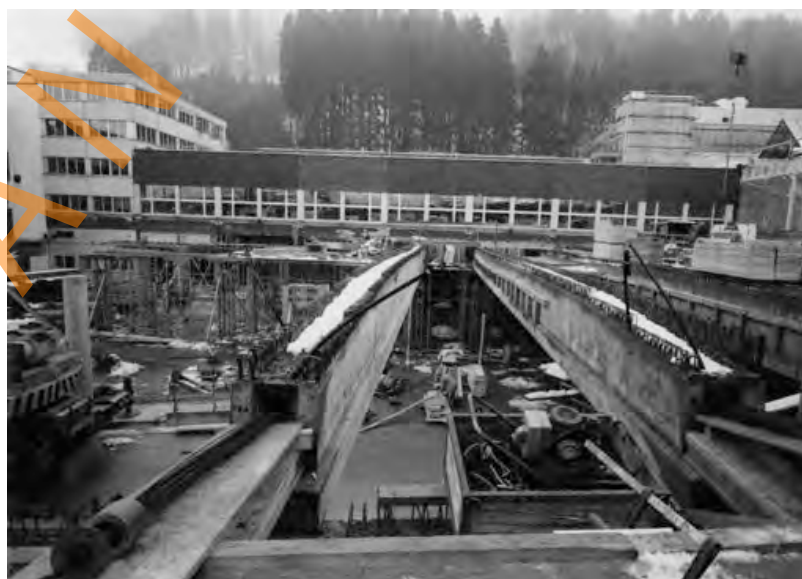
Figure 6.5: Detail of prefabricated beams and prestressing cables during erection stage
