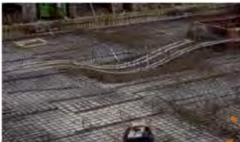
Figure 4.10: Relieving the stresses by means of prestressing cables in the thickened parts of the raft foundation
