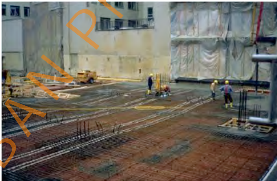
Figure 3.36: Floor slab reinforcement: prestressing cable and top reinforcement
