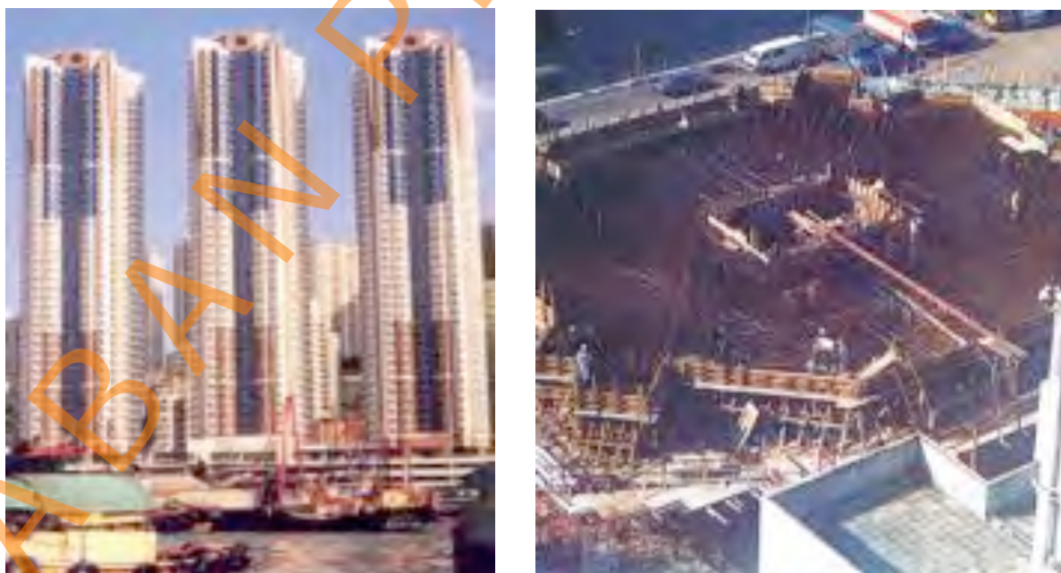
Figure 5.4. a) The three residential blocks facing Aberdeen Harbour, Hong Kong b) View of the transfer plate during the construction
