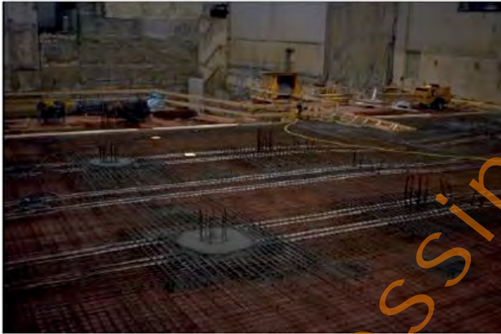
Figure 3.37: Prestressing cable over the columns with pre-concreted concrete plugs made of high strength concrete
