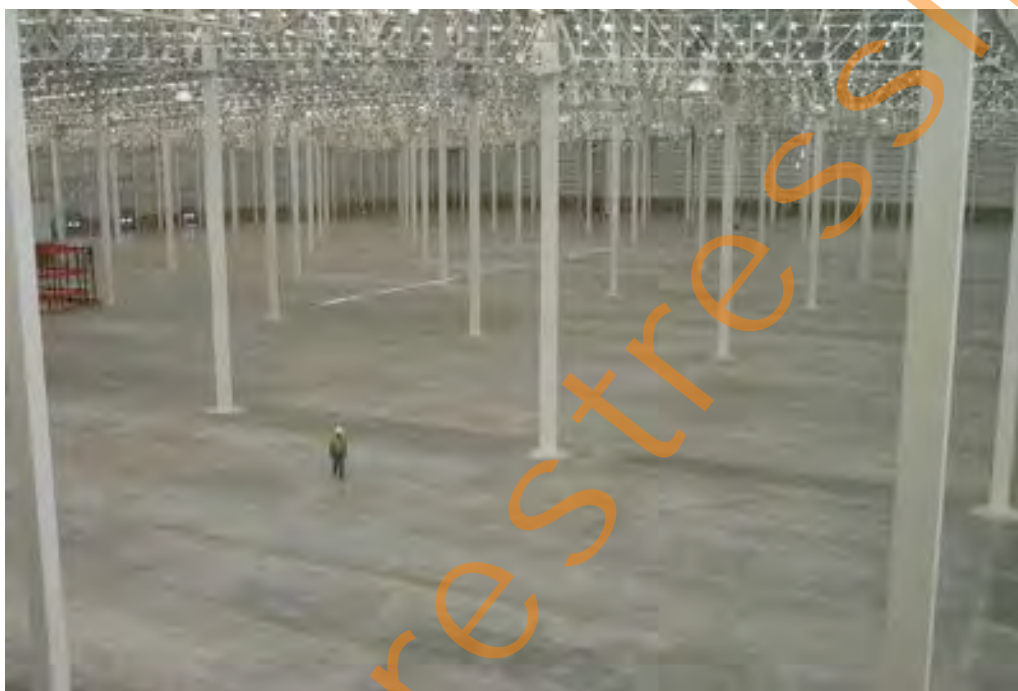
Figure 4.12: Post-tensioning eliminates joint problems for slab on grade floors
