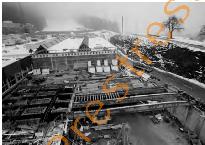
Figure 6.4: Overview of the building site showing areas in situ concrete and the already erected prefabricated beams
