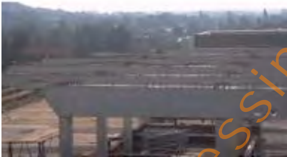
Figure 6.10: Construction stage prefabricated beams placed and fixed
