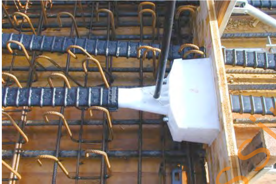
Figure 2.34: Stressing anchorage of group 1
