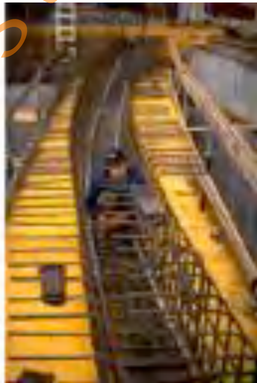
Figure 5.25: Adjustment of the stirrup reinforcement for an opening in the side of the deck slab
