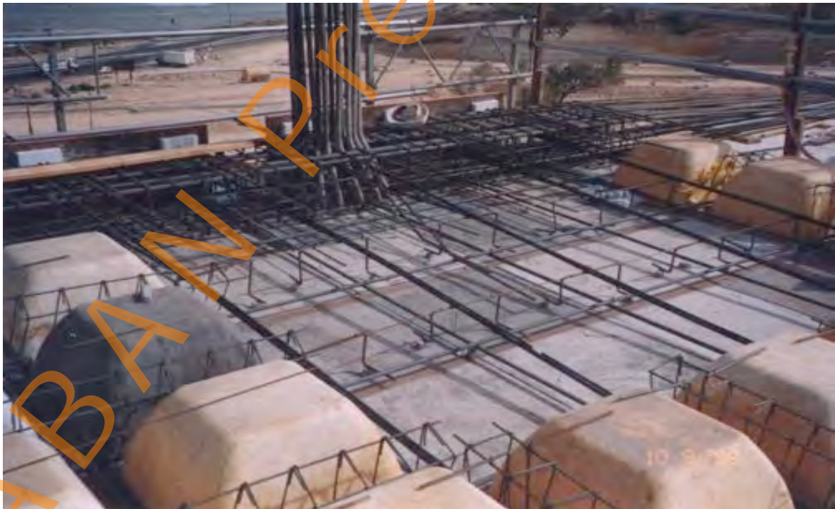
Figure 3.12: View of the waffle slab with single strand cables
