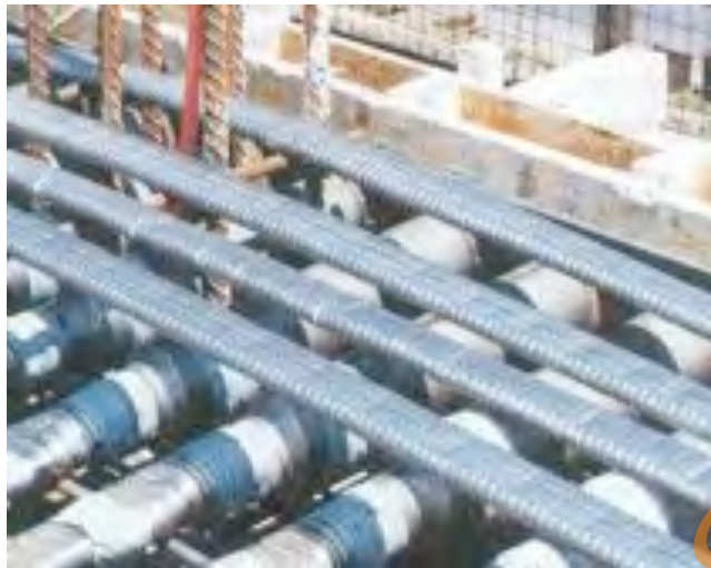
Figure 2.31: Steel flat ducts
