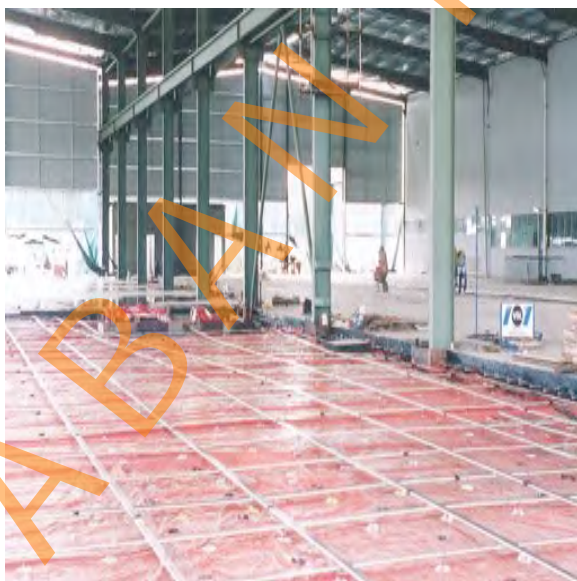
Figure 4.19: View of ground slabs before concreting
