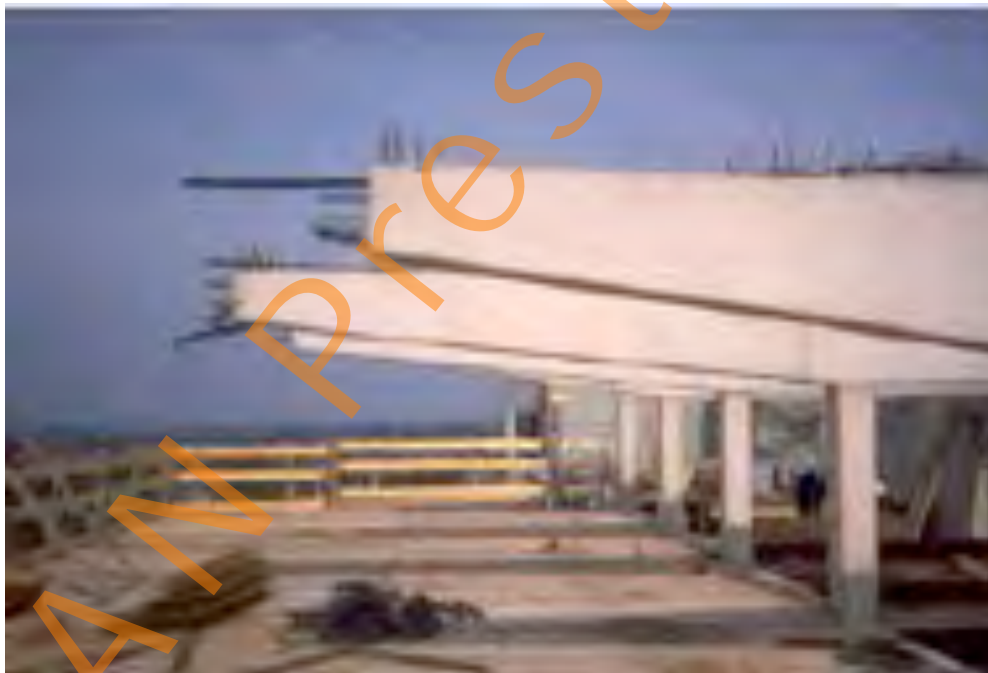
Figure 6.11: Cantilevering prefabricated beams during construction
