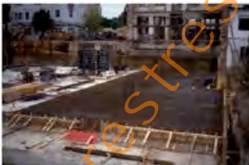
Figure 4.11: Reinforced raft foundation construction stage
